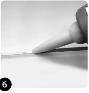
Using appropriate filling material (grout, silicone or mortar) fill down the edges of the Groove Light product into the recessed channel. Ensure that a fair amount of filling material is pushed down the sides of the product and channel to ensure good adhesion.
