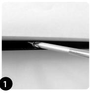
PVC Channel should be secured using suitable fixings for the mounting surface. The PVC Channel can be used to support the entire Groove Light length (Channel length = fitting length), or cut into smaller sections. Minimum 200mm (7.87") of PVC Channel recommended per 500mm (19.69") of Groove Light.
