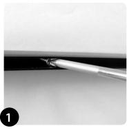
PVC Channel should be secured using suitable fixings for the mounting surface. The PVC Channel can be used to support the entire Groove Light length (Channel length = fitting length), or cut into smaller sections. Minimum 200mm (7.87") of PVC Channel recommended per 500mm (19.69") of Groove Light.
