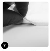
Remove protection mask from the front of the Groove Light product after all sanding, painting and finishing is completed.
