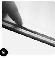
With the Groove Light pushed into the mounting channel, make wiring connections and conceal wiring into recessed channel as required.
